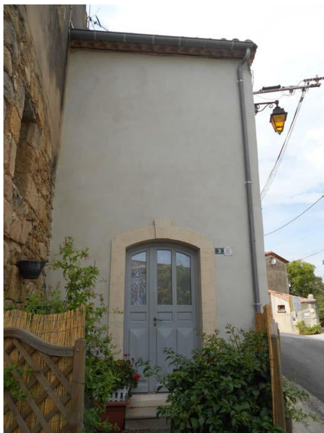
Façade NOE, accolée au Château
